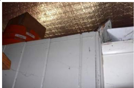
Toilet partition wall, section of skirting missing (left) section of cornice missing, Images: B, T & K Architects 2015
