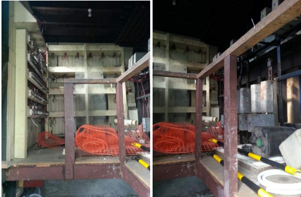
Mezzanine level of the signal box, Images: B, T & K Architects 2015
