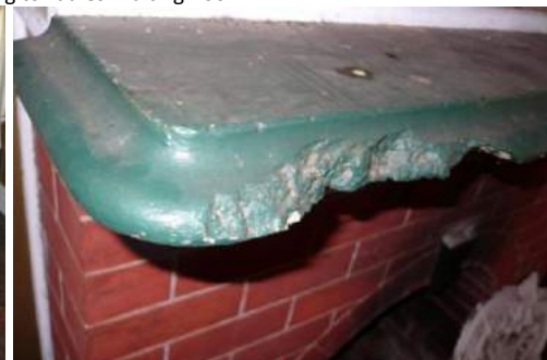
Fireplace on north wall (left) close up of damage to edge of concrete mantle, Images: B, T & K Architects 2015
