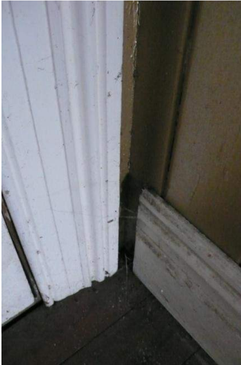
Skirting + architrave junction details
