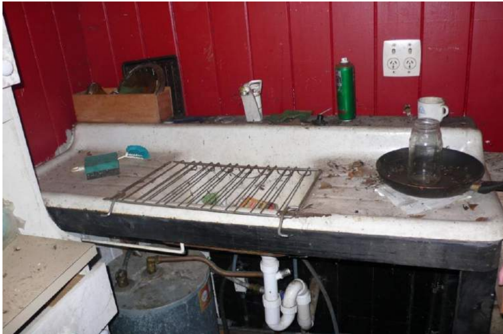
Kitchen sink unit, north wall of kitchen area
