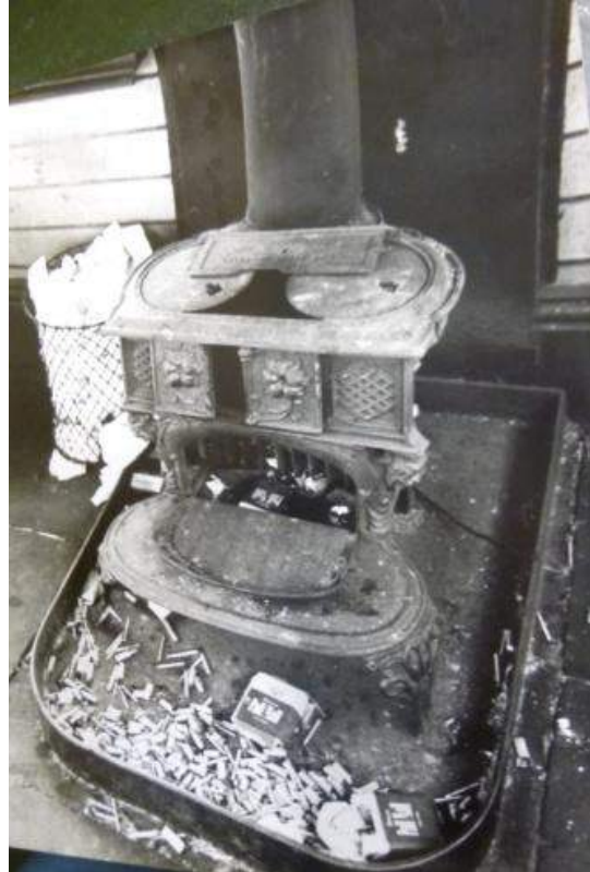
Original wood burning stove in signal box, Image: M.Condon, C.R.Roberts; Measured Drawing Assignment; 1973: Auckland University School of Architecture Library
