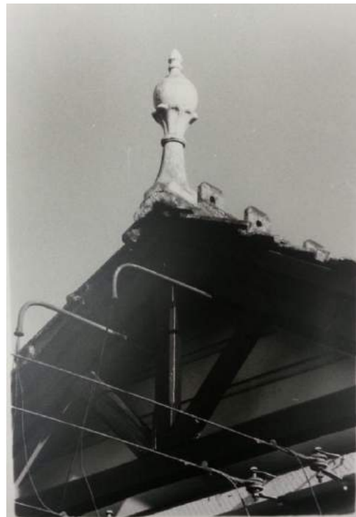
Showing original cast iron finials, spouting & rainwater heads, Image: M. Condon, C. R. Roberts; Measured Drawing Assignment; 1973, Auckland University School of Architecture Library
