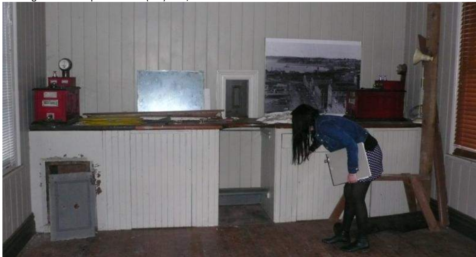
Showing cabinetry, ticket hatch + safe along north wall of Station Master + Booking Office
