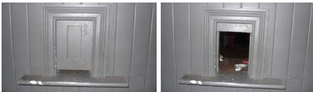
Ticket hatch closed (left) ticket hatch open, Images: B, T & K Architects 2015
