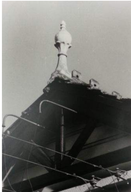
Original finial on the roof of the station building, Image: M.Condon, C.R.Roberts; Measured Drawing Assignment; 1973: Auckland University School of Architecture Library
