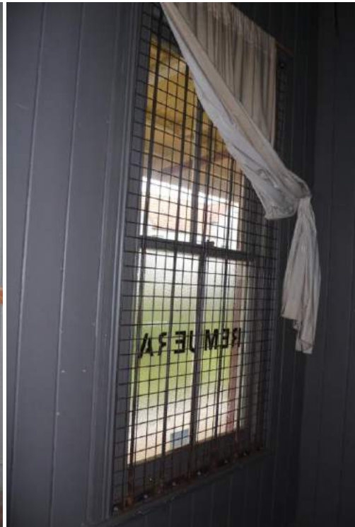
Double doors with locking bar on west wall leading out on to platform (left) wire grills over double hung window
