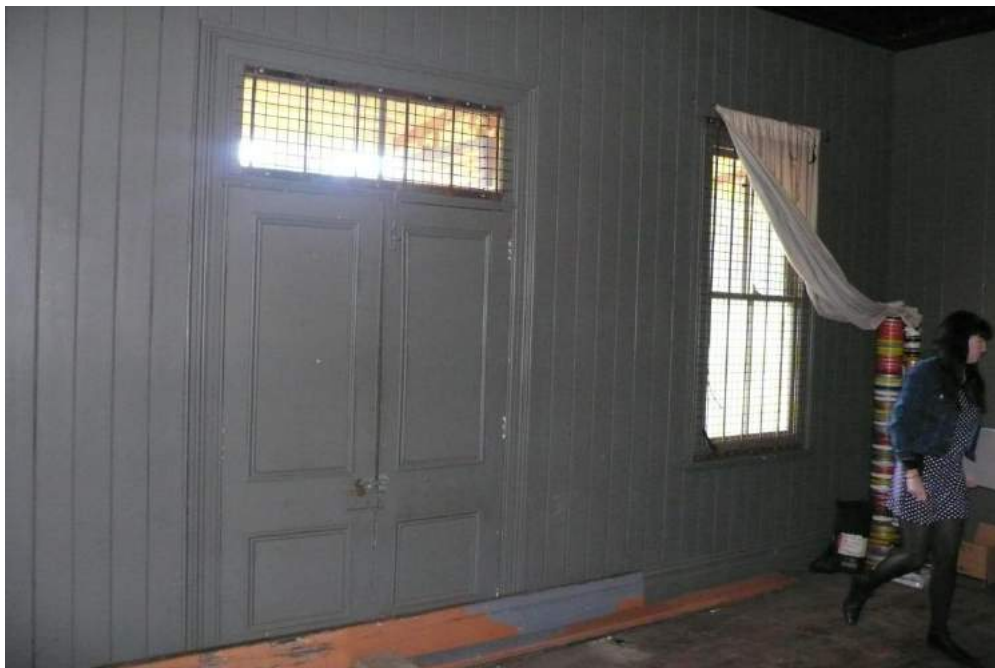
East wall showing double hung window and double doors leading out to platform
