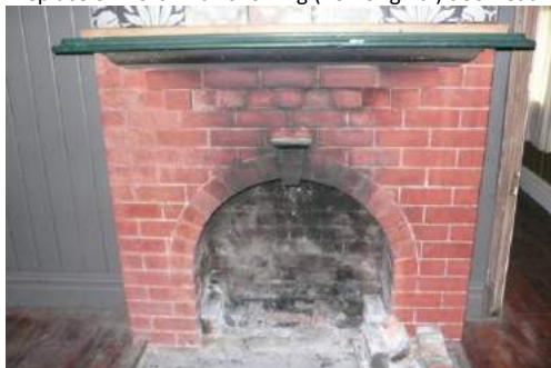
Fireplace on north wall (left) close up of damage to edge of concrete mantle, Images: B, T & K Architects 2015
