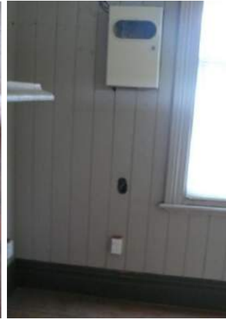
Section of missing skirting board (left) Distribution board on west wall, note hole in t & g lining
