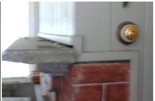
Pressed tin ceiling (left) showing concrete mantle pulling away from wall, Images: B, T & K Architects 2015
