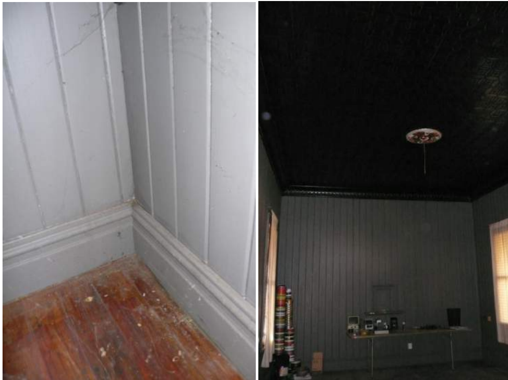
Moulded skirting boards (left) South wall of Public Lobby showing ticket hatch
