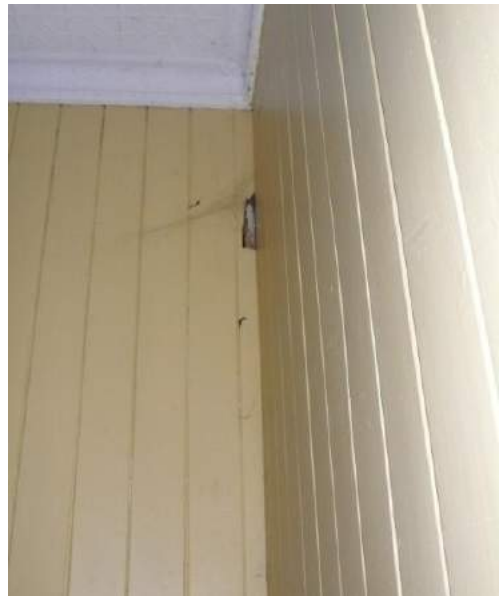
Ceiling rose + hole cut into pressed metal ceiling (left) Damage to t & g wall lining, Images: B, T & K Architects 2015
