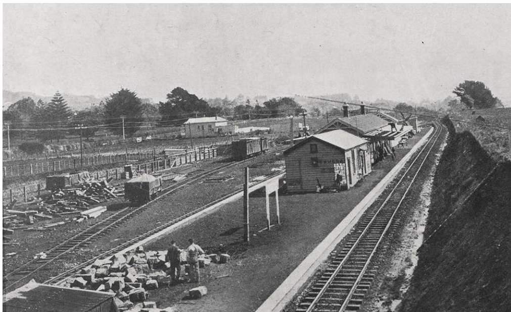
Progress of the Auckland Railway Duplication Works: View of Remuera High-Level Station, showing the Duplicate Lines. 12 September 1907, Image: Sir George Grey Special Collections, Auckland Libraries, Awns-19070912-2-4
