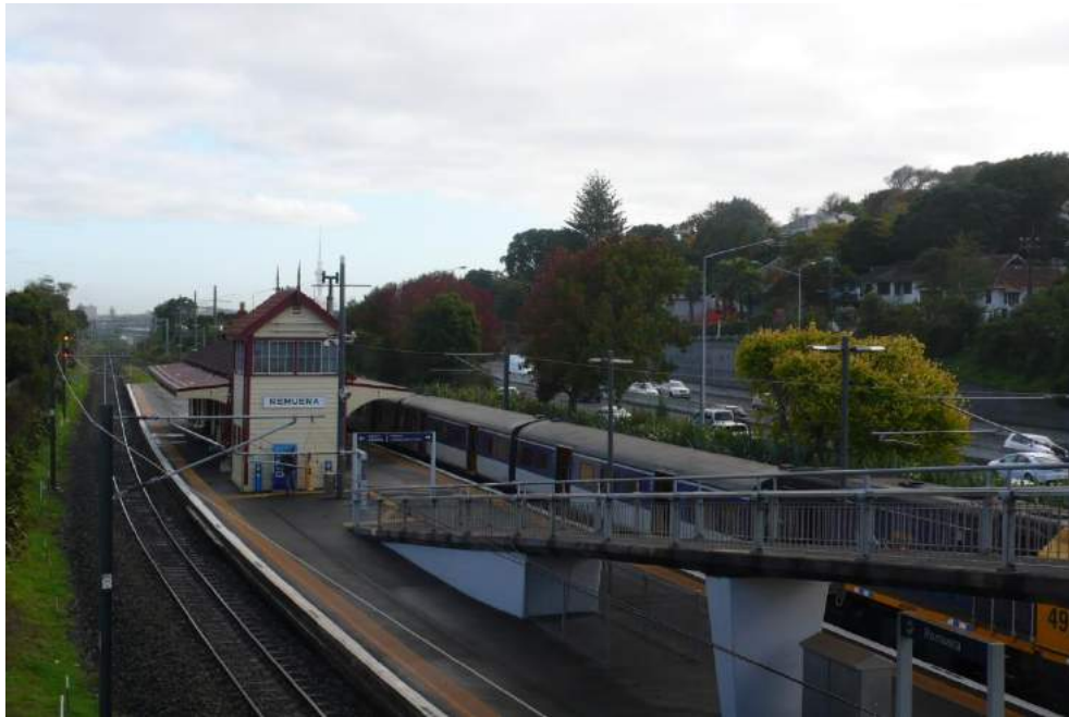
View north from the Market Road Bridge, of the station building and signal box, Image: B, T & K Architects 2015
