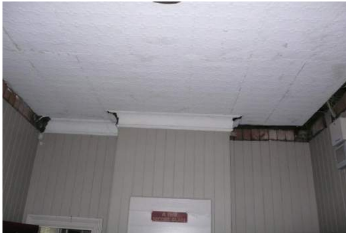
Showing south wall, ceiling with sections of missing cornice (left) missing pressed metal cornice
