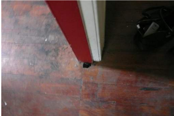
Hole in floor at doorway (left) new doorway into evidence in floorboards of where wall previously ran through
