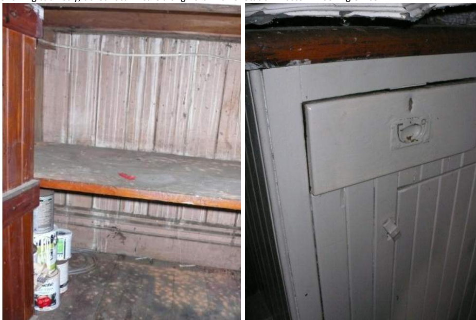
Showing t & g lining to interior of cabinet + evidence of borer (left) cabinetry detail, lockable drawer, Images: B, T & K Architects 2015
