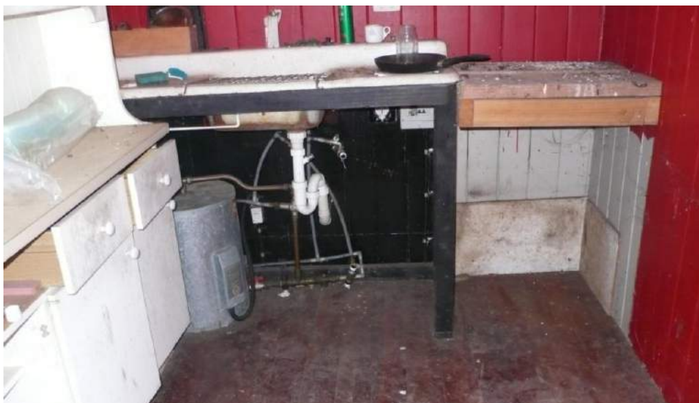
Sink unit along north wall of kitchen area, Images: B, T & K Architects 2015
