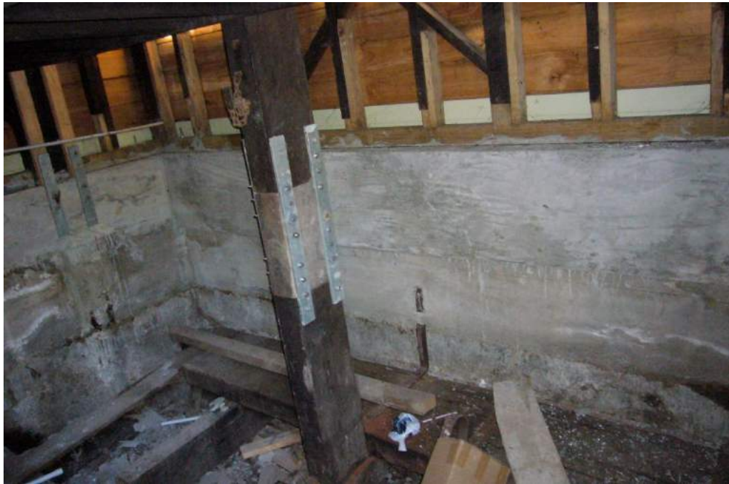
Subfloor of the signal box, Image: B, T & K Architects 2015.
