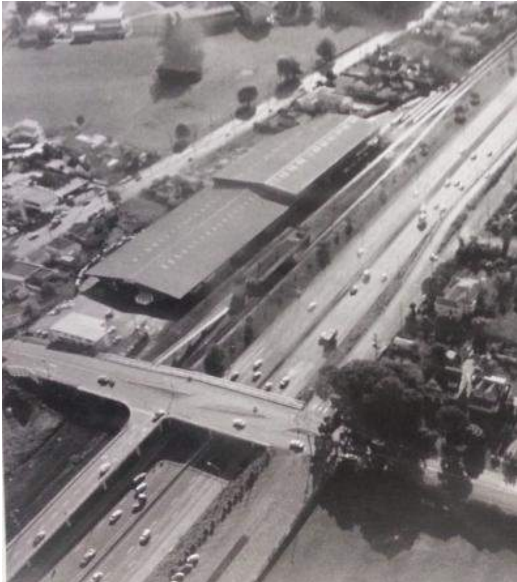
Rail Sheds (demolished) c. 1970s, Image: M. Condon, C. R. Roberts; Measured Drawing Assignment; 1973, Auckland University School of Architecture Library
