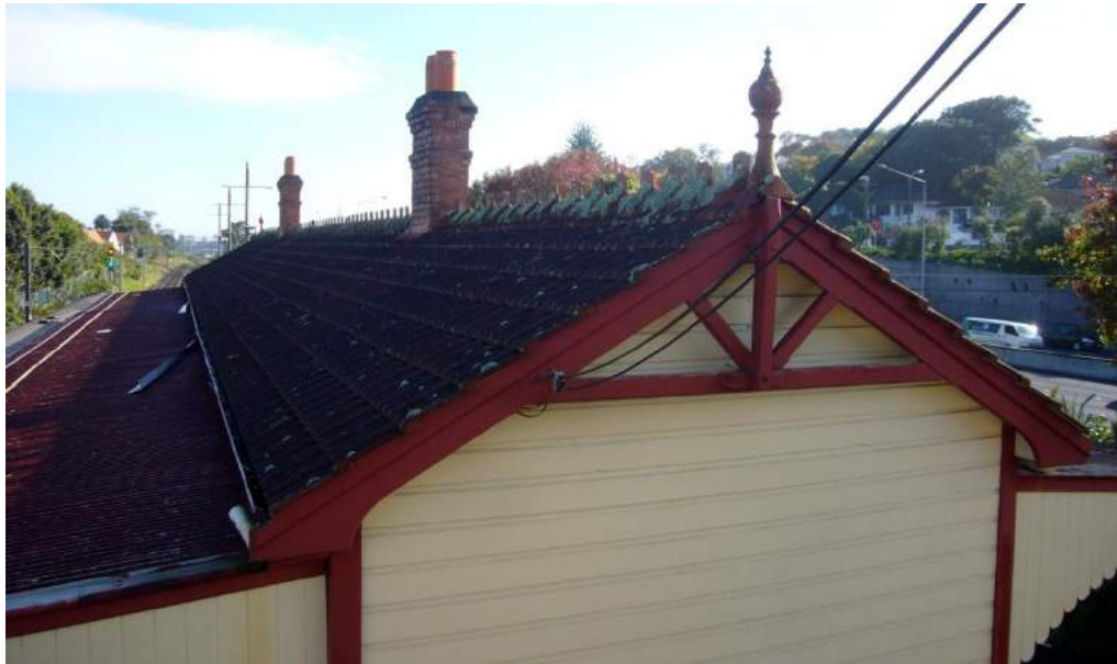
Roof of the Station Building, Image: B, T & K Architects 2015.
