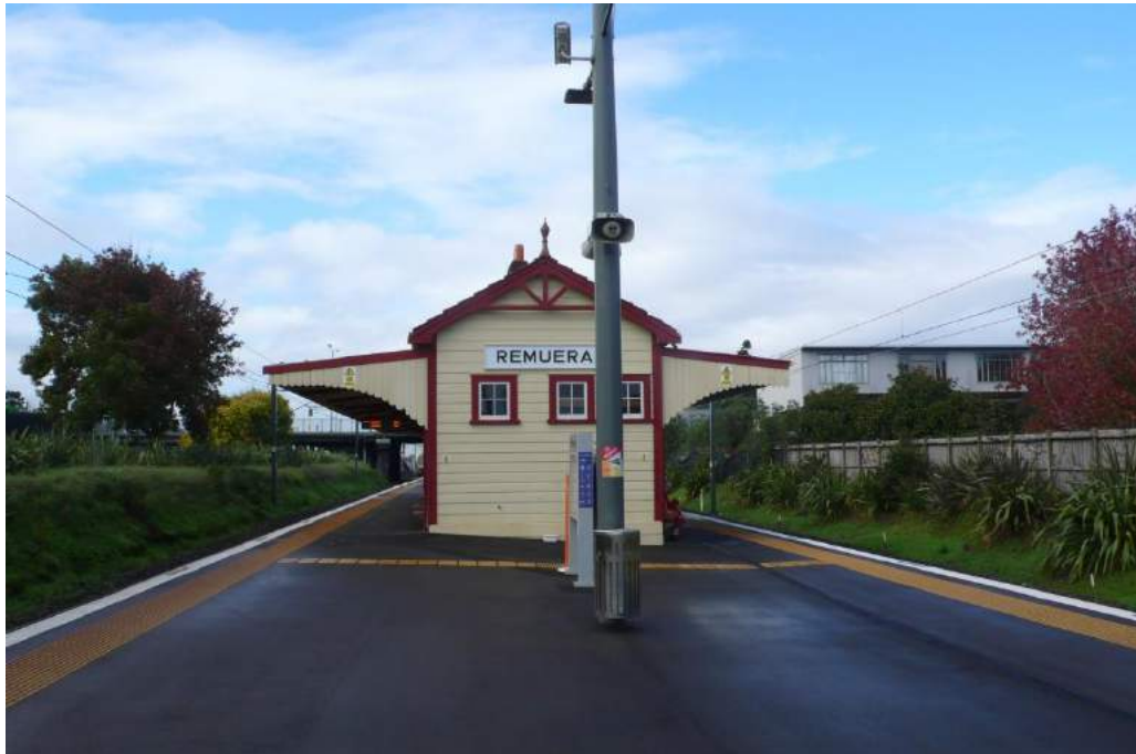
North elevation of the station building, Image: B, T & K Architects 2015
