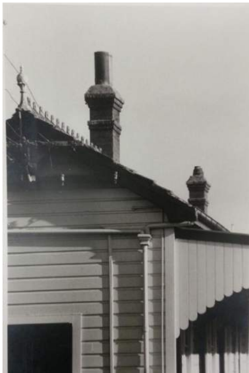
Showing original cast iron finials, spouting & rainwater heads, Image: M. Condon, C. R. Roberts; Measured Drawing Assignment; 1973, Auckland University School of Architecture Library
