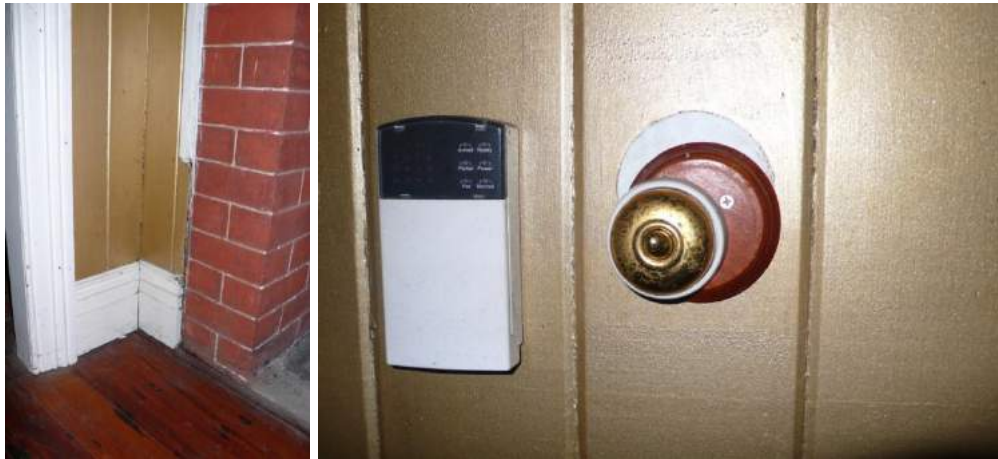
Skirting, wall & fireplace junction (left) light switch & security alarm system
