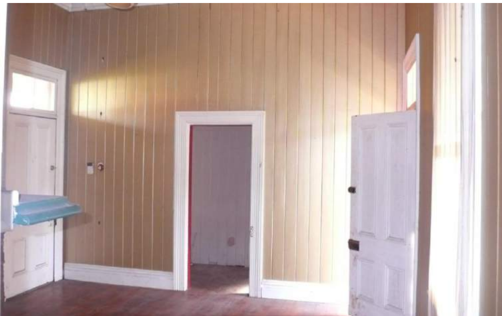
North wall of ladies waiting showing door through to kitchen/ bathroom, Image: B, T & K Architects 2015
