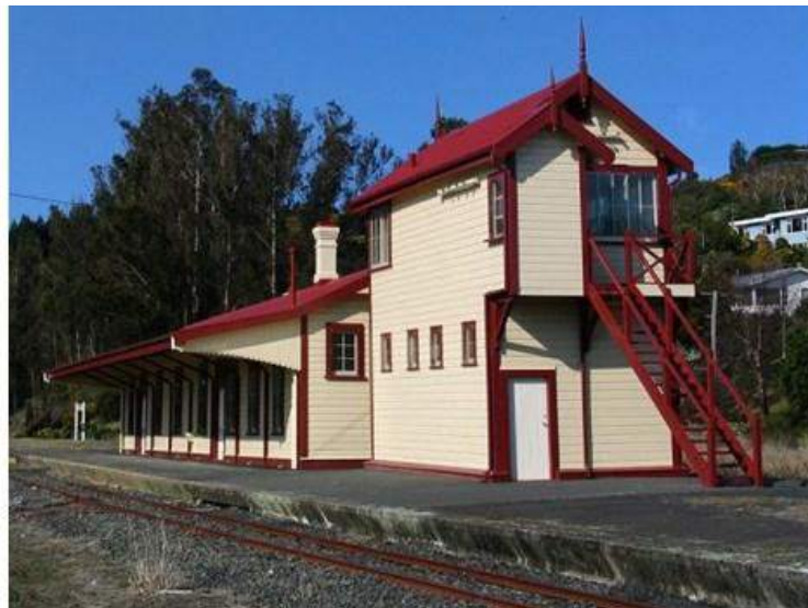
Wingatui Railway Station Signal Box.
