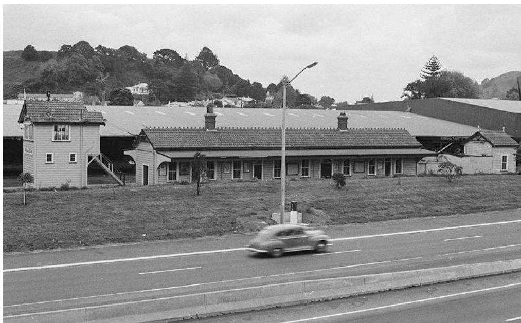
Remuera railway station, viewed from across motorway, Image: MOTAT; Les Downey; 1973; 14-2501
