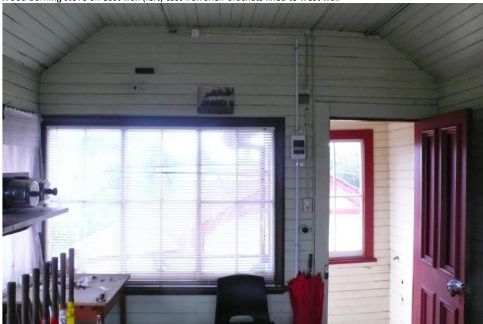
North wall showing door to exterior
