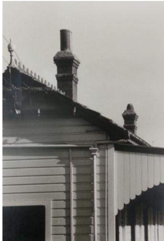
Showing original cast iron spouting, downpipes and rainwater heads. Image: M. Condon, C. R. Roberts; Measured Drawing Assignment; 1973: Auckland University School of Architecture Library
