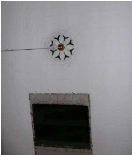
Ceiling rose + hole cut into pressed metal ceiling (left) Damage to t & g wall lining, Images: B, T & K Architects 2015
