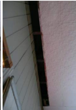
Showing south wall, ceiling with sections of missing cornice (left) missing pressed metal cornice
