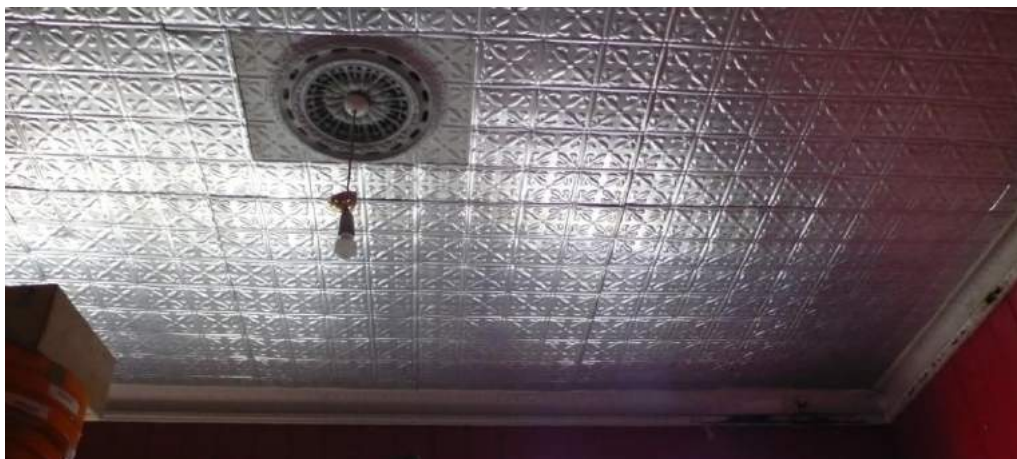
Showing new pressed metal ceiling in kitchen area + ceiling rose, Image: B, T & K Architects 2015
