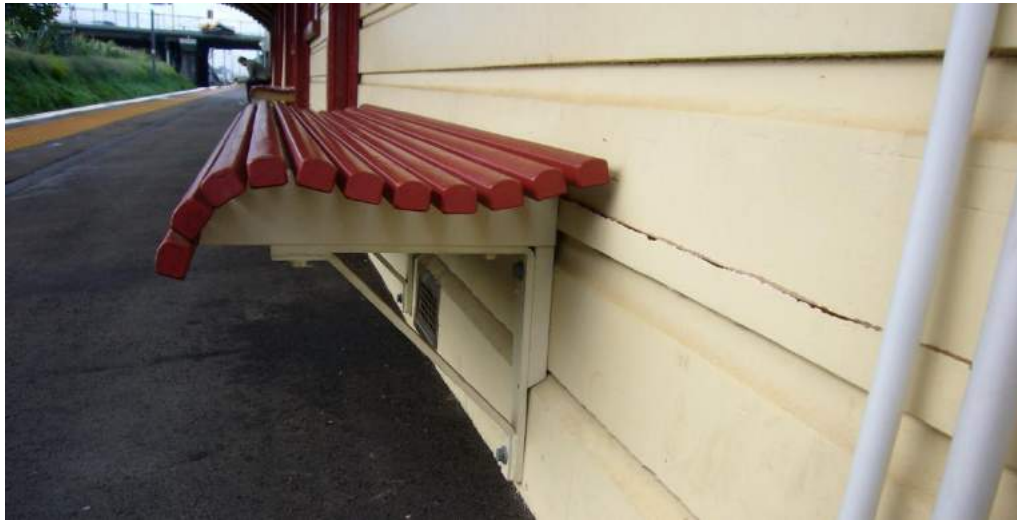
Timber slatted seats, Image: B, T & K Architects 2015.
