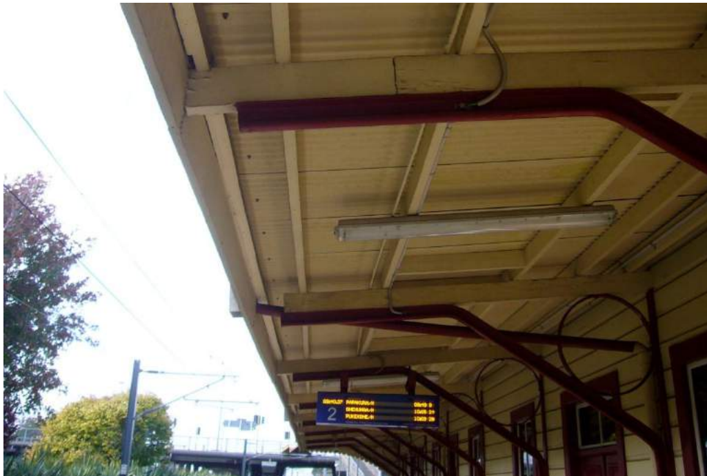
Showing the underside of the station verandah roof, Image: B, T & K Architects 2015.
