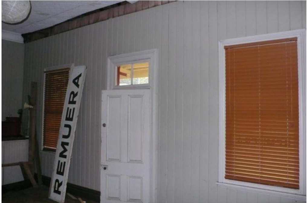
Eastern wall of Station Master & Booking Office showing door leading out to platform and sign leant up against wall Images: B, T & K Architects 2015
