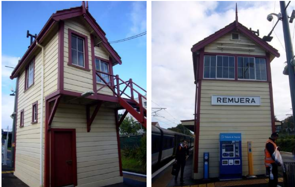
Showing the north east corner (left) and southern facade of the Signal Box, Images: B, T & K Architects 2015
