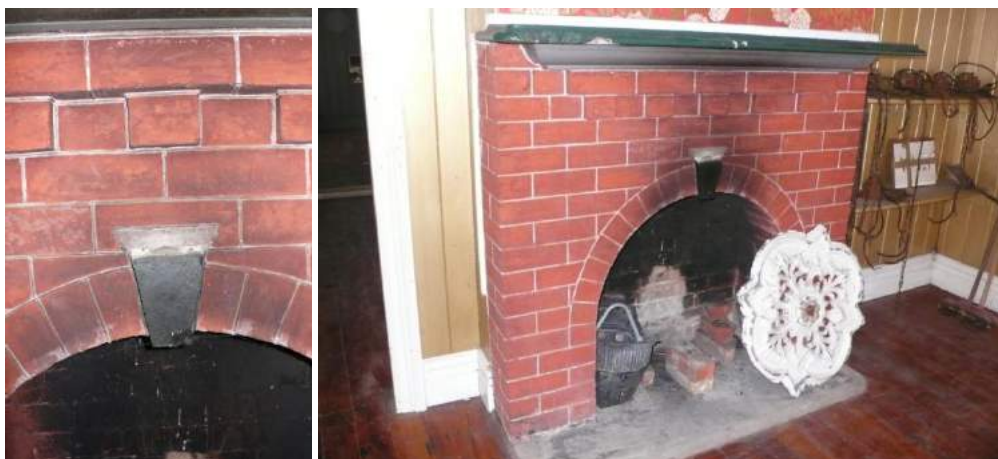
Detail of fireplace (left) Fireplace with concrete mantle in southern wall, Images: B, T & K Architects 2015
