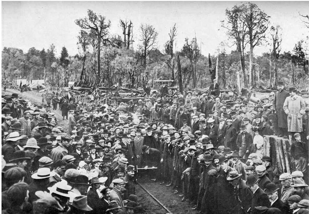
On 6 November 1908 Prime Minister Joseph Ward ceremonially opened the North Island main trunk line by driving in a final polished silver spike at Manganuioteao, between National Park and Ohakune. Image: http://www.nzhistory.net.nz/media/photo/final-spike-nimt
