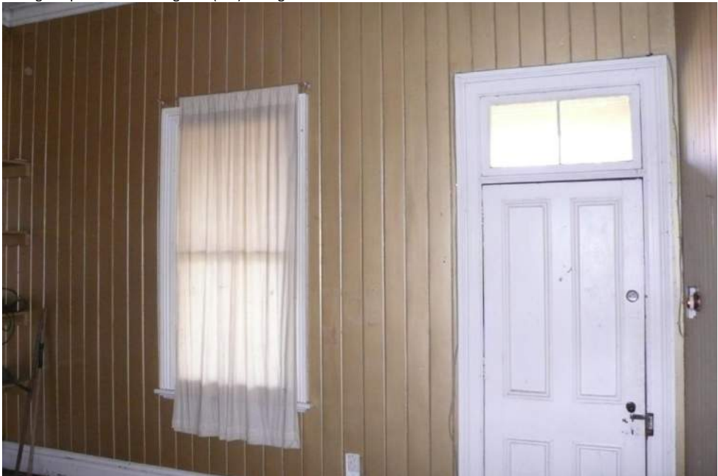
Western wall of Ladies Waiting, Images: B, T & K Architects 2015
