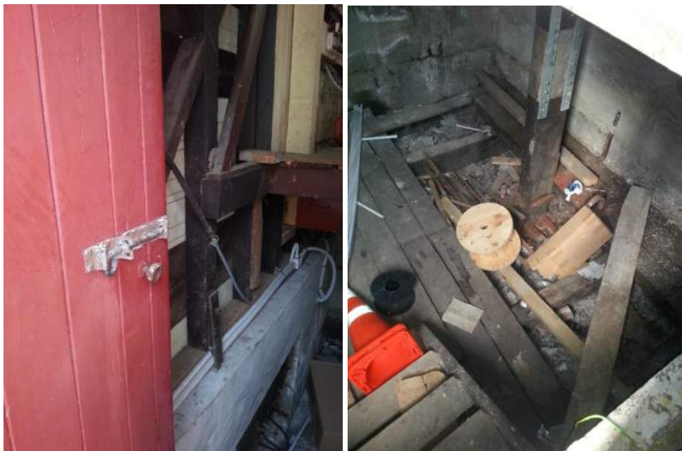
Exterior door to signal box, lower level (left) subfloor of the signal box, Images: B, T & K Architects 2015
