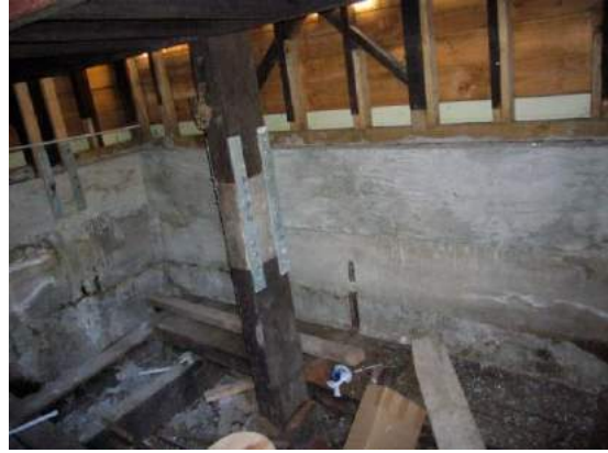
Subfloor of the signal box, Image: B, T & K Architects 2015.
