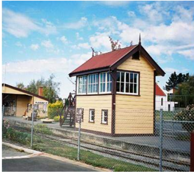
Signal Box (Part of Railway Museum).
