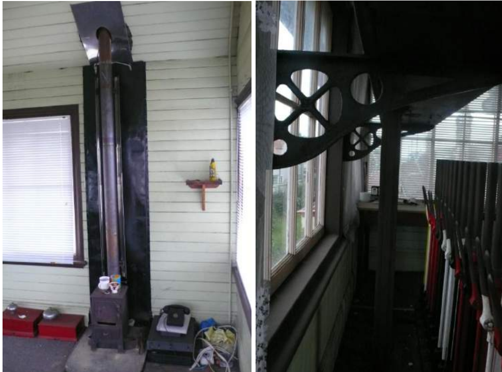
Wood burning stove on east wall (left) cast iron shelf brackets fixed to west wall
