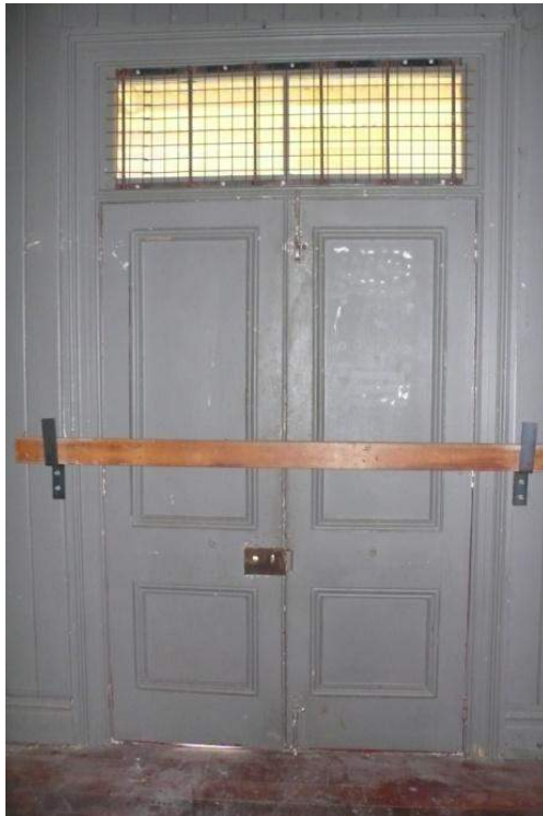
Double doors with locking bar on west wall leading out on to platform (left) wire grills over double hung window
