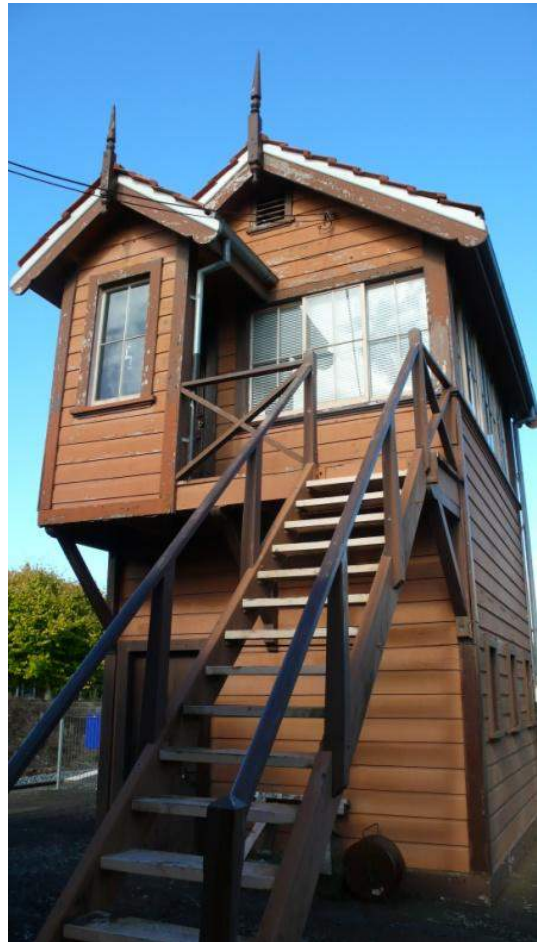
Showing paint colour scheme on the signal box c. 2003, Image: B, T & K Architects 2015.
