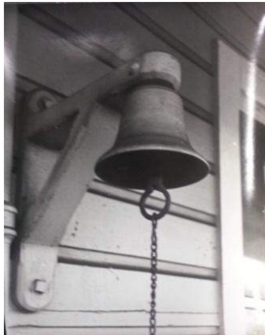
Original bell fixed to station wall on timber bracket, Image: M. Condon, C. R. Roberts; Measured Drawing Assignment; 1973: Auckland University School of Architecture Library
