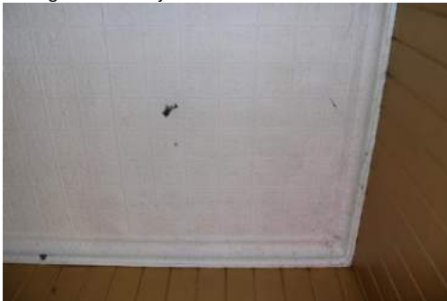
Damage to pressed tin ceiling tiles (left) ceiling rose
